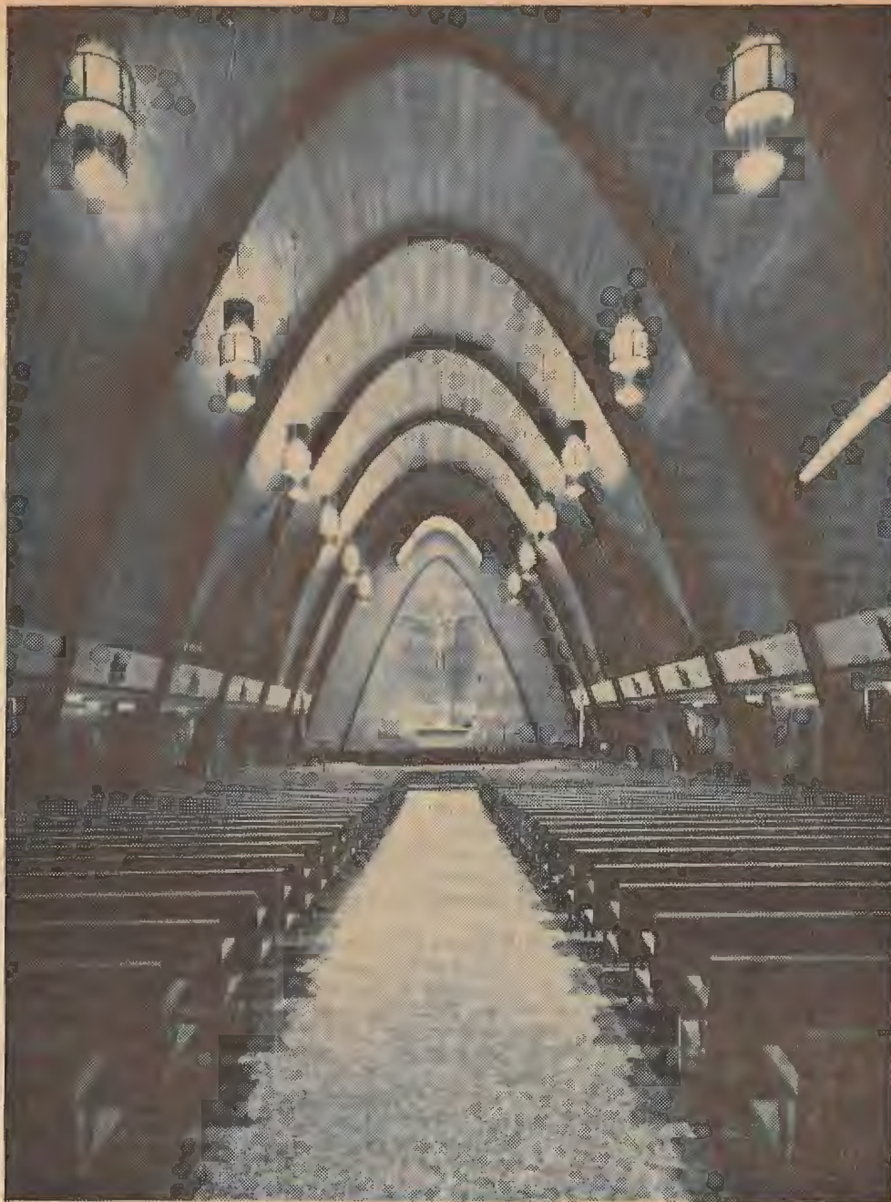
PHOTO COURTESY OF UNIT STRUCTURES, INC.
