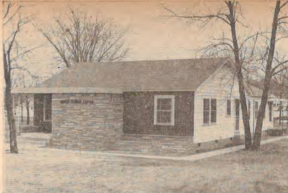
ADDITION OF a new front to the Arkansas Tech Student Center has given the building an appearance of being wider. Boston siding with redwood stain finish is used to blend with the pinkish ledgerstone and with the red bricks, which will be used later in veneering the remainder of the building. Gerald Stone, now serving as pastor of McKay Mission, Little Rock, drew the plans. Mr. Stone is a former Tech student who was an architectural major at the University.
