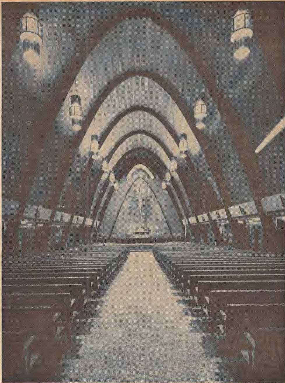
PHOTO COURTESY OF UNIT STRUCTURES, INC.
