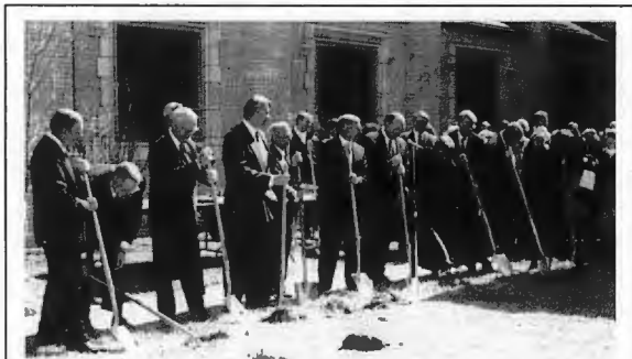
Breaking ground March 10 for a $3.5 million building project for First Church of Blytheville are (left to right) building committee chairman Pat Sullivan, pastor Bill Fuller, architect Muriel Lewis, building contractor Doug Henson, trustee Jim Gardner, chairman of deacons Bill Sullivan, church training director Gary Hollis, Woman's Missionary Union director Marvel Dickerson, Baptist Men's president Edwin Holstead, building finance committee chairman Dick Trout and youth council representative Abigail Hubbard. Fuller said the congregation is "traveling new roads of opportunity for reaching new people for Jesus Christ and for discipling people" as they begin the 54-week building program which will feature a chapel, office complex and family life center. Church members pledged $1.61 million for the project during a recent "Together We Build" fund-raising campaign. The building project also includes remodeling the present fellowship hall into educational space.
