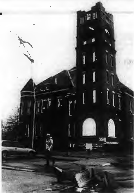
▲ The historic Clark County courthouse shows the impact of the tornado that ravaged downtown Arkadelphia. The storm damaged the building's windows, roof and clock tower.
