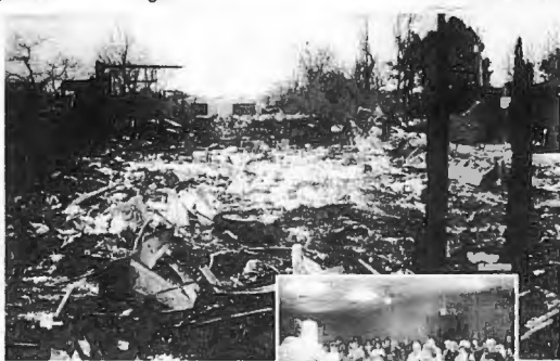
Westside Church in Warren (above) burned into the morning of Jan. 18 as a result of a heater malfunction. The next Sunday members met for worship services at a nearby rented sanctuary (inset).
