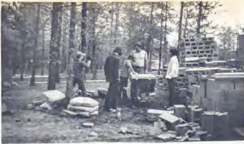
As construction started.
