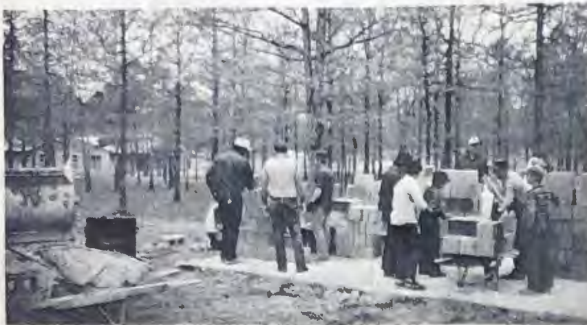
The first blocks are in place.
