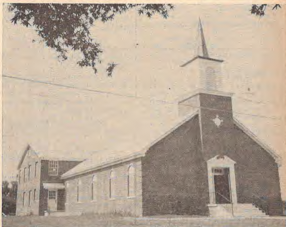
FIRST CHURCH, Hampton, has improved the appearance and usefulness of their building with a remodeling program. Pastor C. Phelan Boone came to the church May 25 from Tinsman Church.
