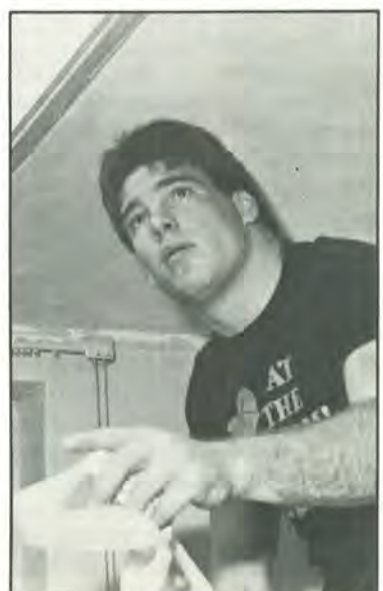
■ A Red Shirt member repairs a ceiling.
