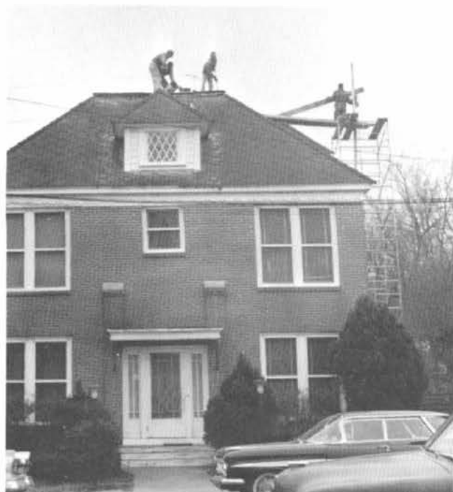
Workmen repair the roof on the Home Management Building.
