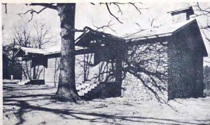
Union Valley Church meets in this new building.
