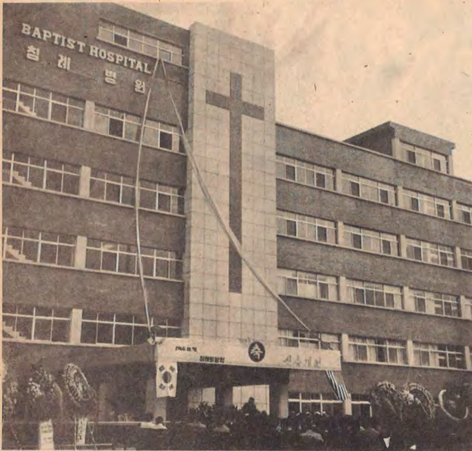
STREAMERS, flags and floral wreaths decorate the new six-story, 150-bed Wallace Memorial Baptist Hospital building in Pusan, Korea, during dedication services on Oct. 30. The hospital, named for the late Dr. William L. Wallace, missionary to China, was constructed with Lottie Moon Christmas Offering funds.
