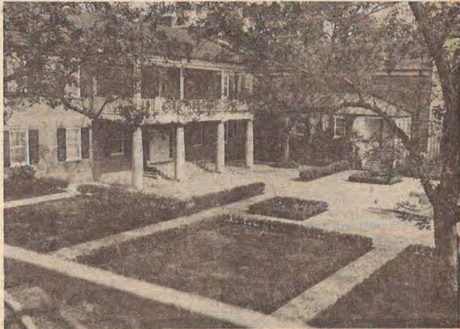
EARLY LOUISIANA ARCHITECTURE prevails at New Orleans Seminary as revealed by Mississippi Alumni Garden and the J. M. Frost Religious Education Building.
