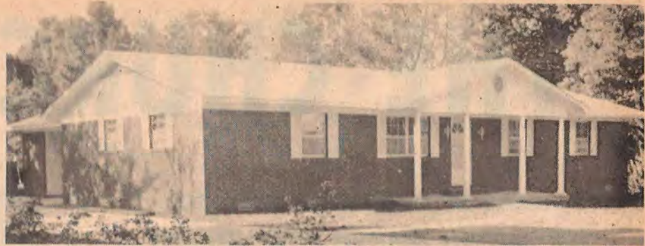
NEW PARSONAGE, First Church, Beebe, was recently completed at a cost of $21,500. The building committee members were Marvin Fisher, chairman, Euell Adams, Roy Showalter, Daisy Fisher, Grace Crouch, and Vernon Cole. Walter N. Hill is pastor.
